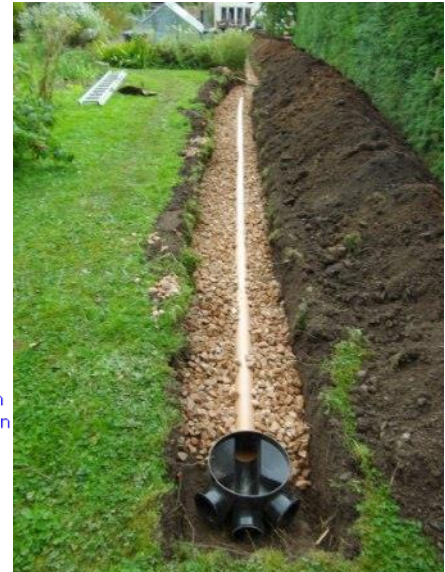
Figure 2.21 – Soakaway scheme (www.pavingexpert.com, 2015)
