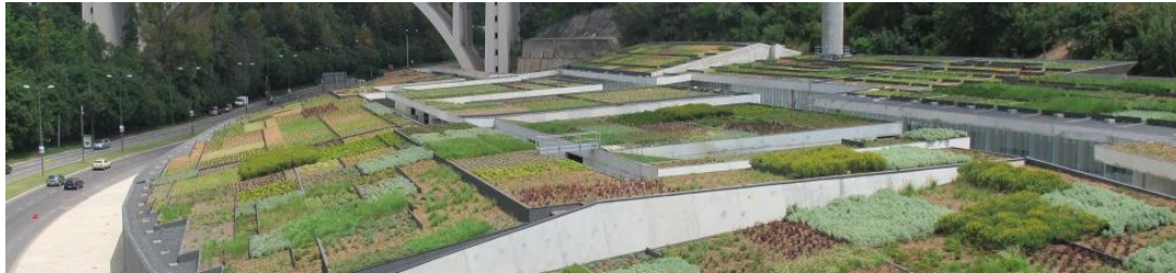
Figure 2.12 - Green roof in ETAR de Alcântara, Portugal
