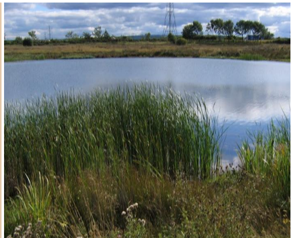
Figure 2.25 - Retention pond (Susdrain, 2015)
