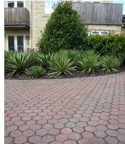
Figure 2.10 – Permeable pavement (Susdrain, 2015)
