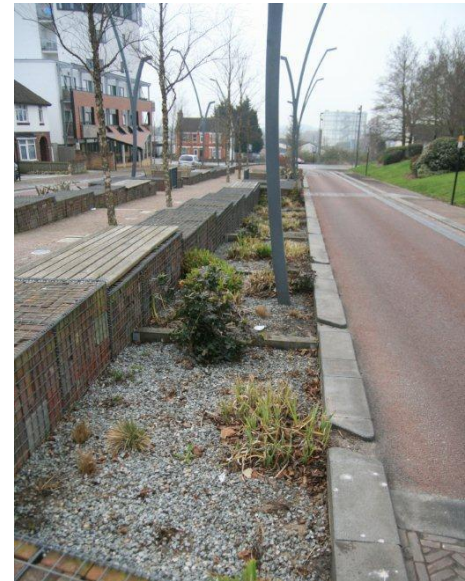
Figure 2.19 - Bioretention area (2015)
